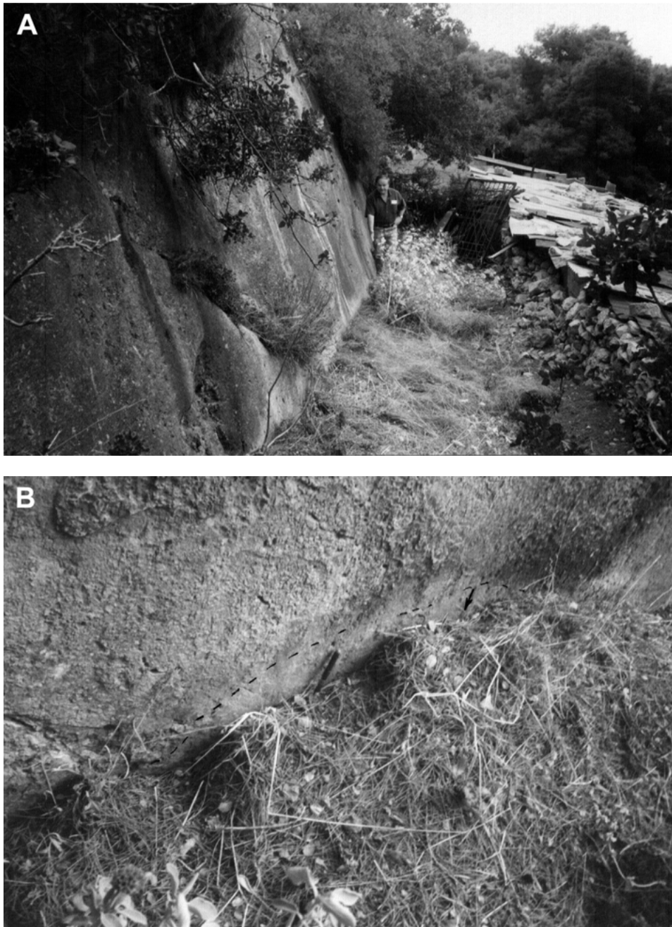
Figure 8. Field photographs. (a) polished fault surface and light band (site 3b in Figure 1, Fili fault) and (b) a possible co-seismic or triggered by the shock displacement along the same fault plane.
