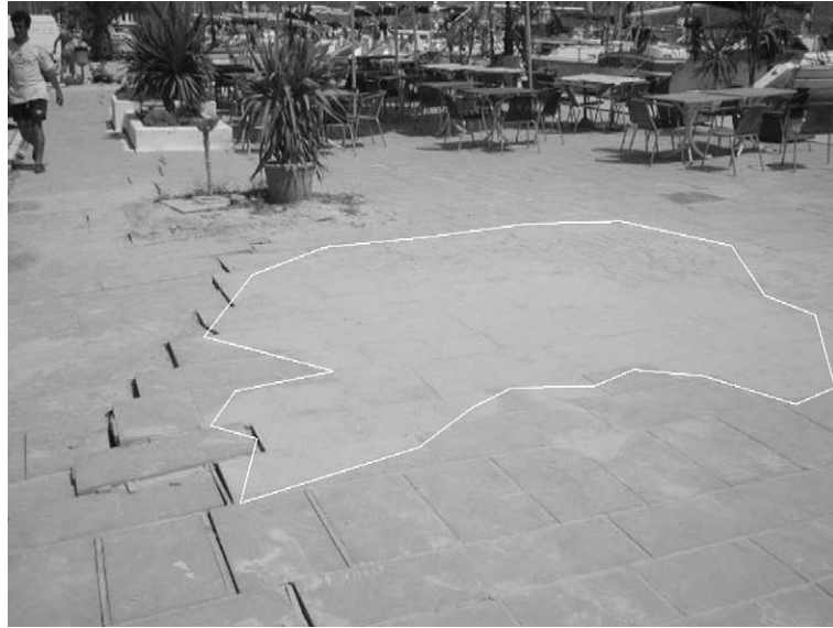
Fig. 17. Ejected sand from fissures in the pavement of the seaside in the town of Lefkada, sampleID: LEF2 (photo taken by Papathanassiou, 15/08/2003).
