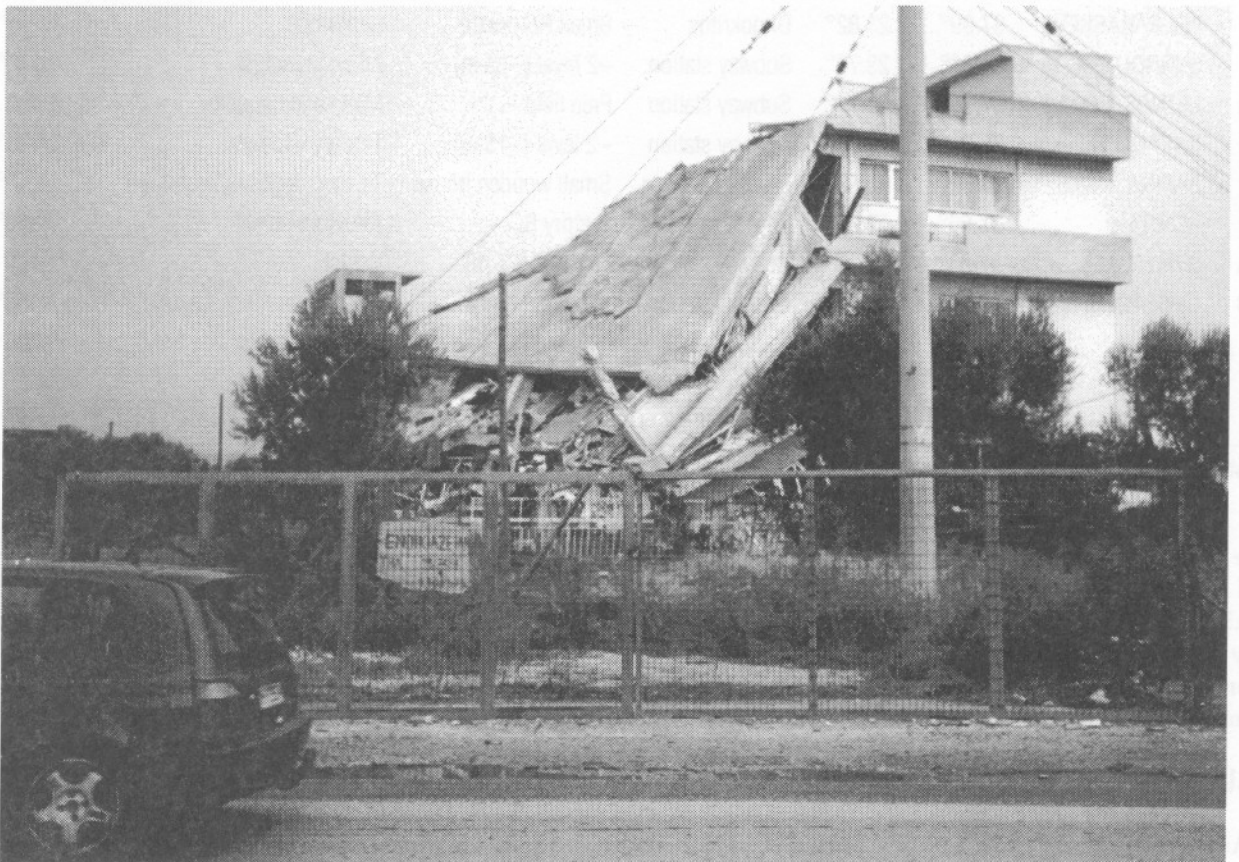
▲ Figure 6. Partial collapse of a three-story house in Aharnes.
