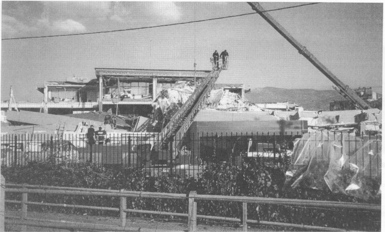
▲ Figure 5. Rescue operation at the Fourlis factory installation in Kato Kifisia, the front part of which collapsed.
