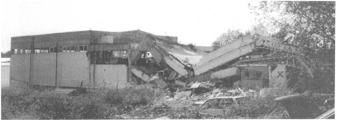
▲ Figure 7. Partial collapse of a small two-story factory installation in Aharnes.
