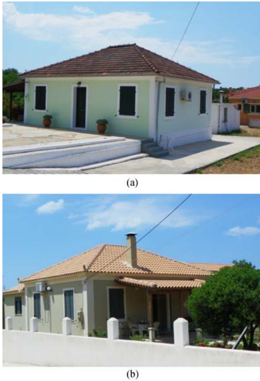
Fig. 12 Two “Arogi Houses” - condition of both as was after the earthquake. (a) As built (b) with lateral extension to the left, through a URM addition
