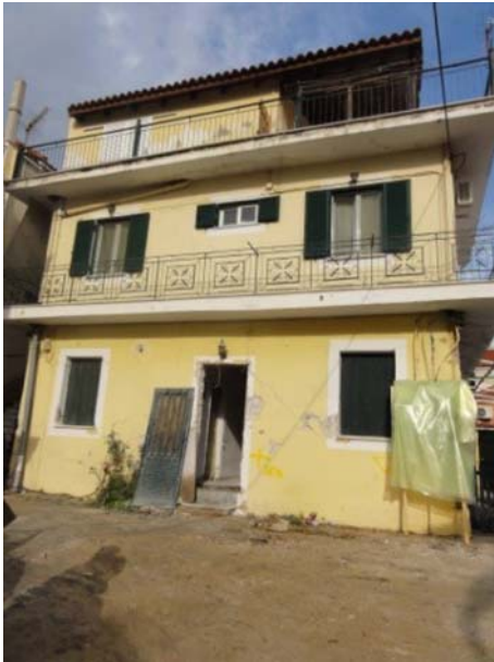
Fig. 13 Extension in height with the addition of a reinforced concrete frame
