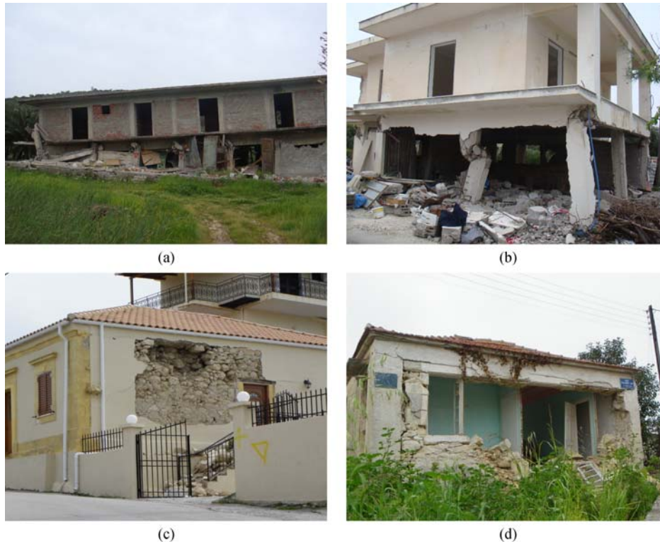
Fig. 2 Seismic damage due to the 2014 Cephalonia Earthquake, (a) and (b) recently constructed R.C. buildings with notable deficiencies non-conforming to the established code practices, (c) and (d) in URM buildings built prior to the big earthquake of 1953
