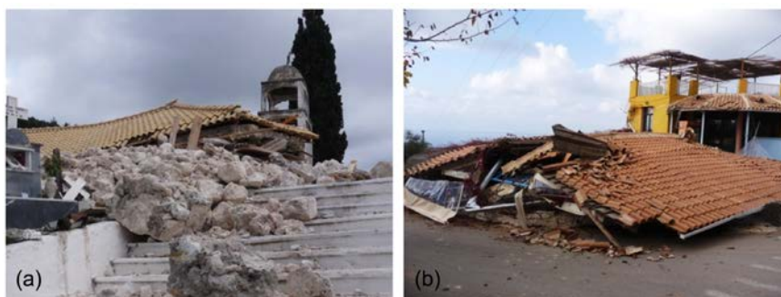
Figure 9. (a) Collapsed church of Agia Paraskevi in Athani; (b) Collapsed kiosk near Athani.
