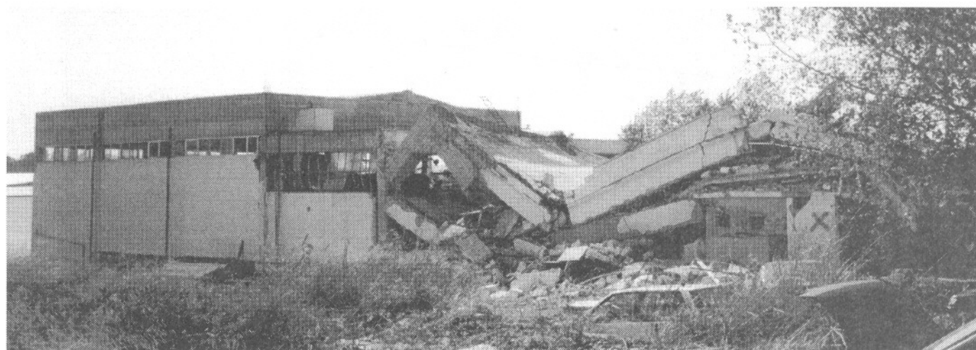
▲ Figure 7. Partial collapse of a small two-story factory installation in Aharnes.
