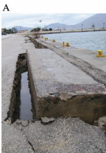
Figure 14. Failures observed at the dock of the Lixouri port after the third strong earthquake of 3.2.2014. Extensive cracking and subsidence (A) and artificial embankment material ejected from a dock crack due to liquefaction (B).
