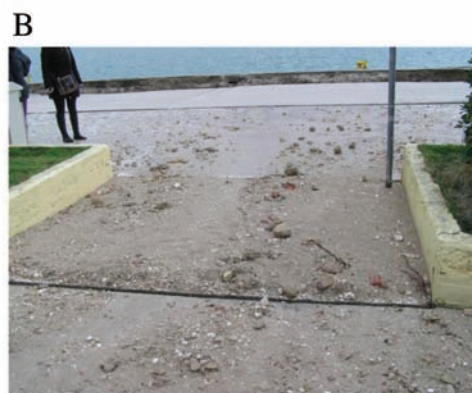
Figure 14. Failures observed at the dock of the Lixouri port after the third strong earthquake of 3.2.2014. Extensive cracking and subsidence (A) and artificial embankment material ejected from a dock crack due to liquefaction (B).
